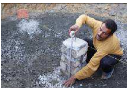
Picture 4 Construction of central pillar
