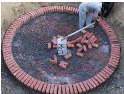
Picture 7 Laying of first layer of bricks
