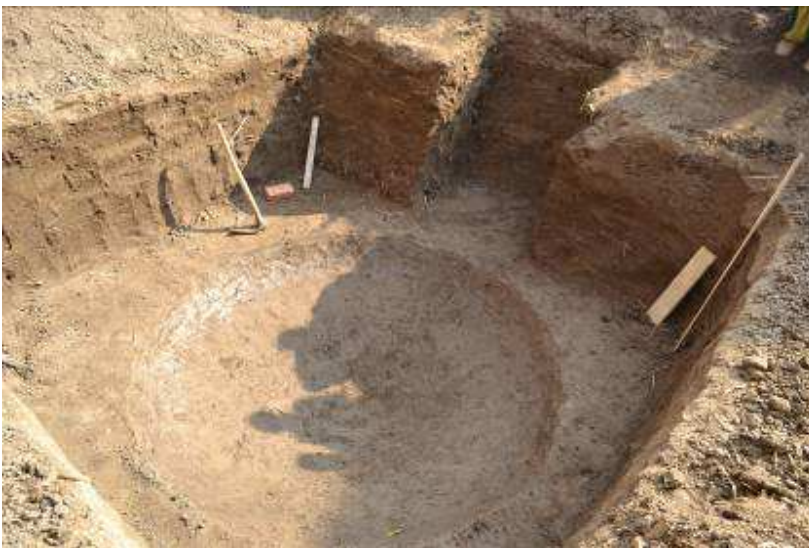
Picture 2 A trimmed pit ready for floor concrete
