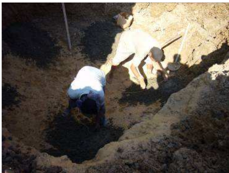
Picture 3 Using a simple level to ensure a horizontal floor
