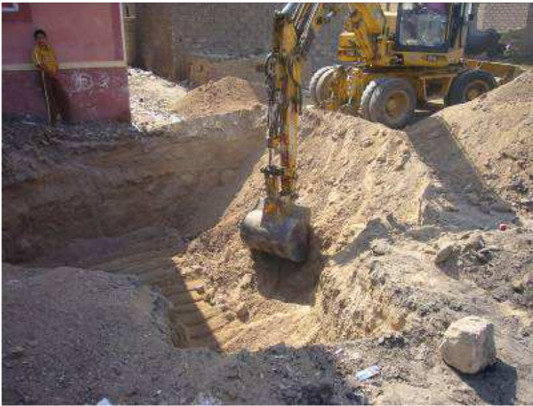
Picture 1 Excavation of a pit for plant installation using machine
