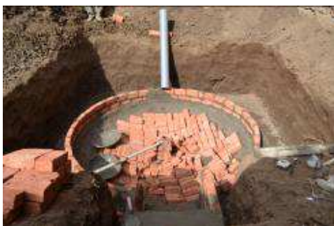
Picture 10 Placing of inlet pipe
