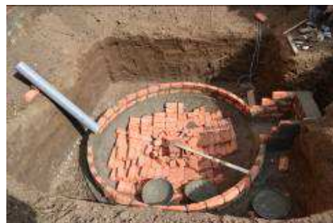
Picture 11 Fitting of inlet pipe
