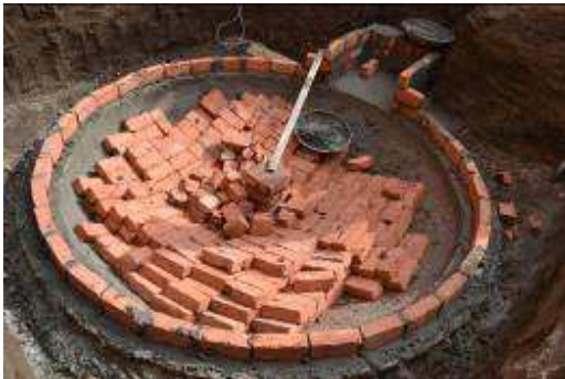
Picture 9 starting construction of the digester
