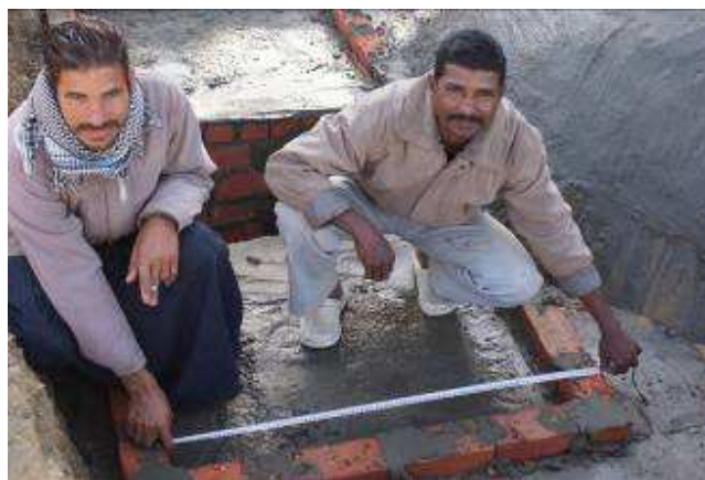
Picture 17 Bricks have to correctly placed
