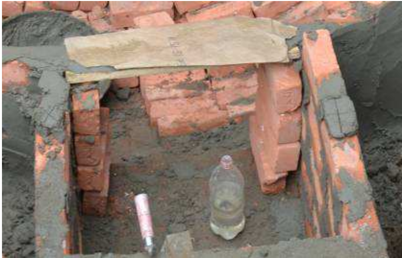
Picture 14 Support plank for box tank ceiling layer
