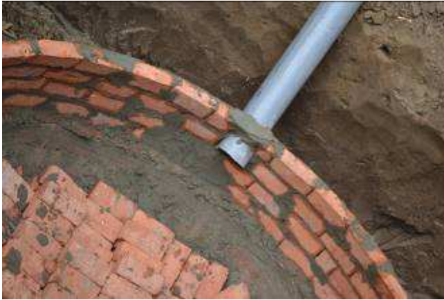
Picture 12 Fixing of inlet pipe
