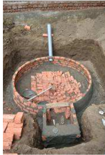
Picture 13 Alignment of inlet pipe
