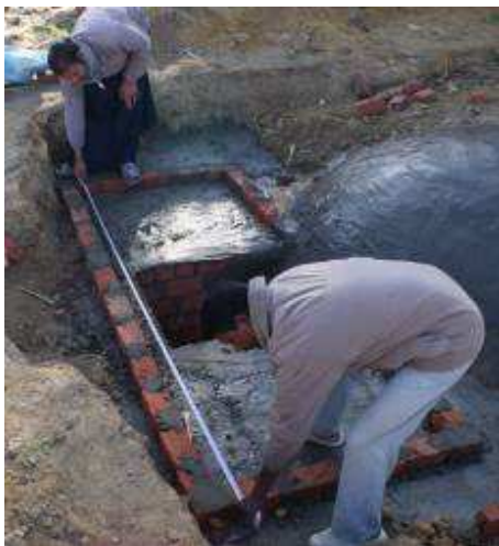
Picture 16 First layer of bricks
