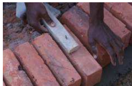
Picture 8 Spacing first layer of bricks
